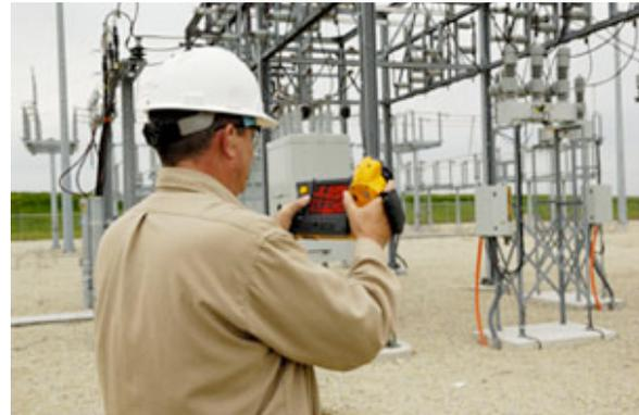
Predictive Maintenance means that maintenance is performed on troublesome equipment just before it fails. Therefore, PdM relies heavily on Condition Monitoring (CM) of the equipment and systems. Included in the Monitoring processes are the application of the available technologies and how they're used. The basic technologies are vibration levels and signature analysis, oil analysis (spectroscopy), infrared thermography, and acoustics.
